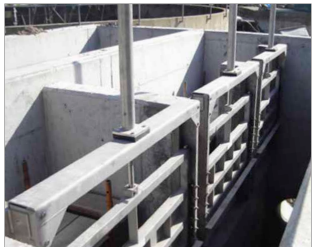
Tilting Weir – Allows control of upstream water levels by means of a weir plate fixed to an operating shaft. The weir plate seals off side cheeks and rotates through a 90°. The tilting weir is specified when there is insufficient levels beneath invert to permit a conventional weir Penstock.
