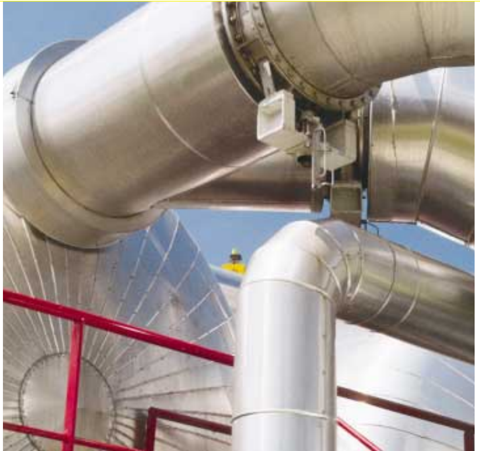
Actuator with hydraulic speed control
